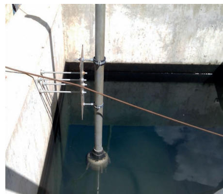
Sonatax sc probe over sludge collection hopper.
